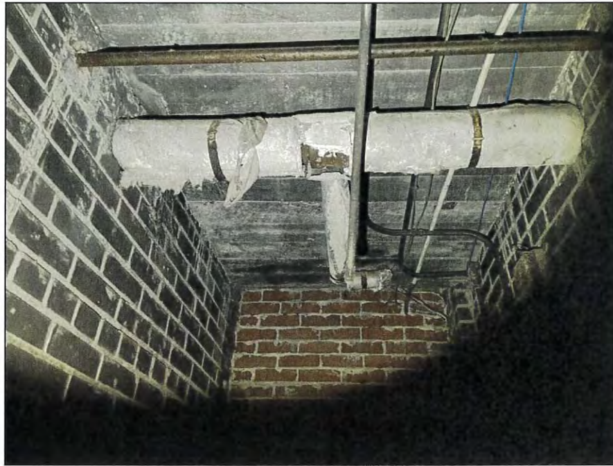
7 - ACM Damaged Boiler Room Pipe Insulation
