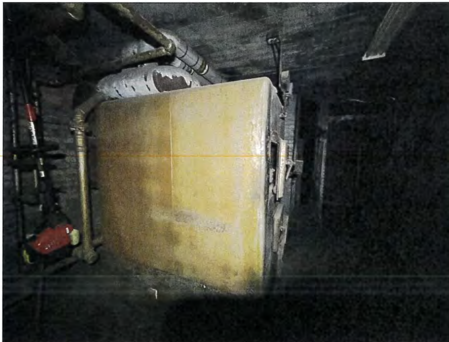
8 - Boiler Assumed to Contain ACM Insulation in Walls and Doors
